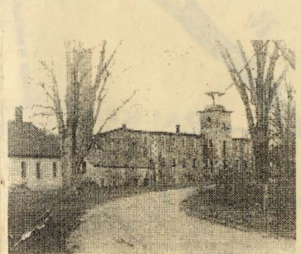
View looking east (toward Plainfield) showing the 1832 stone textile mill.
